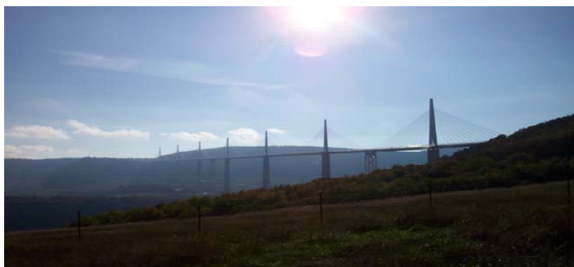
Figure 4: Verrières Viaduct (north of Millau Viaduct)
