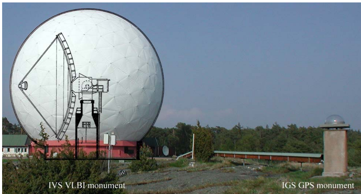
Figure 1: Equipment for space geodetic observations at the Onsala Space Observatory. Left: The radome enclosed 20 m radio telescope used for geodetic VLBI (IVS monument). Right: The permanently installed and radome equipped antenna used with Global Navigation Satellite Systems (GNSS) (IGS monument). The two monuments are located within about 80 m distance.
