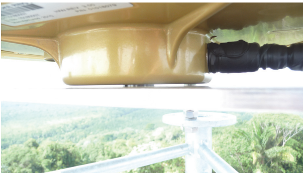
Figure 6: Left) Example of antenna deficiency (AR25)
