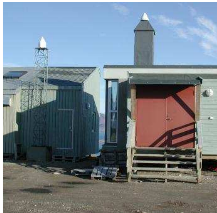
Figure 2: GPS antennas NYA1 (right) and NYAL (left).
